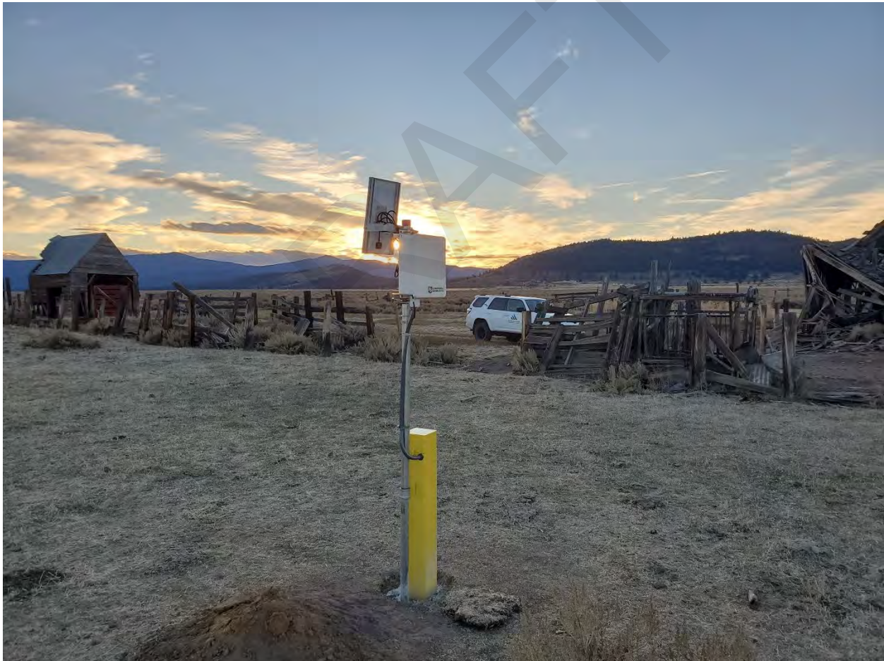
Photograph showing completed GDE piezometer installation at GDE Site 4.
