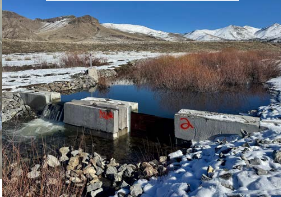
Recharge Check Structure near Staverville Creek
